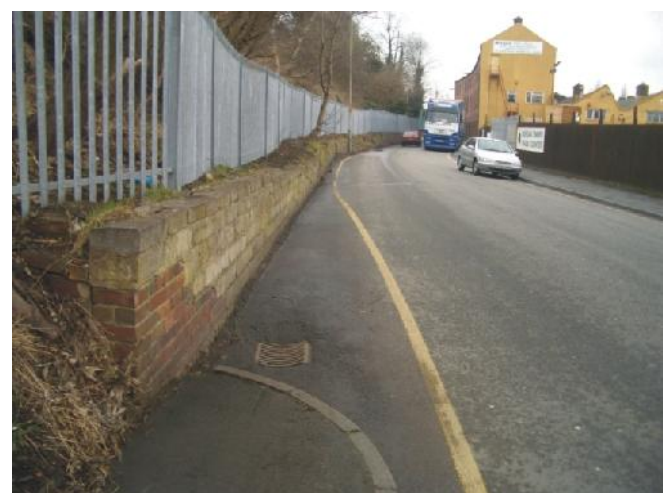
Photo 6.9 - Retaining wall of variable height and quality. End of footpath on west side of Park Lane.
