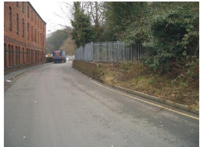
Photo 6.3 - Park Lane to the south of the Rock Works with base of ramped access to wooded greenspace on the right
