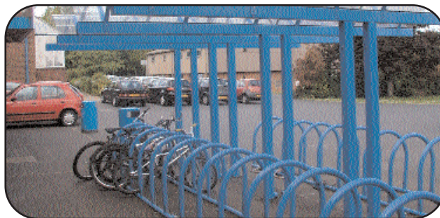
Covered Cycle Parking at Harry Cheshire High School, Kidderminster.
