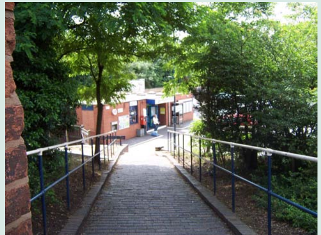
Kidderminster Rail Station
