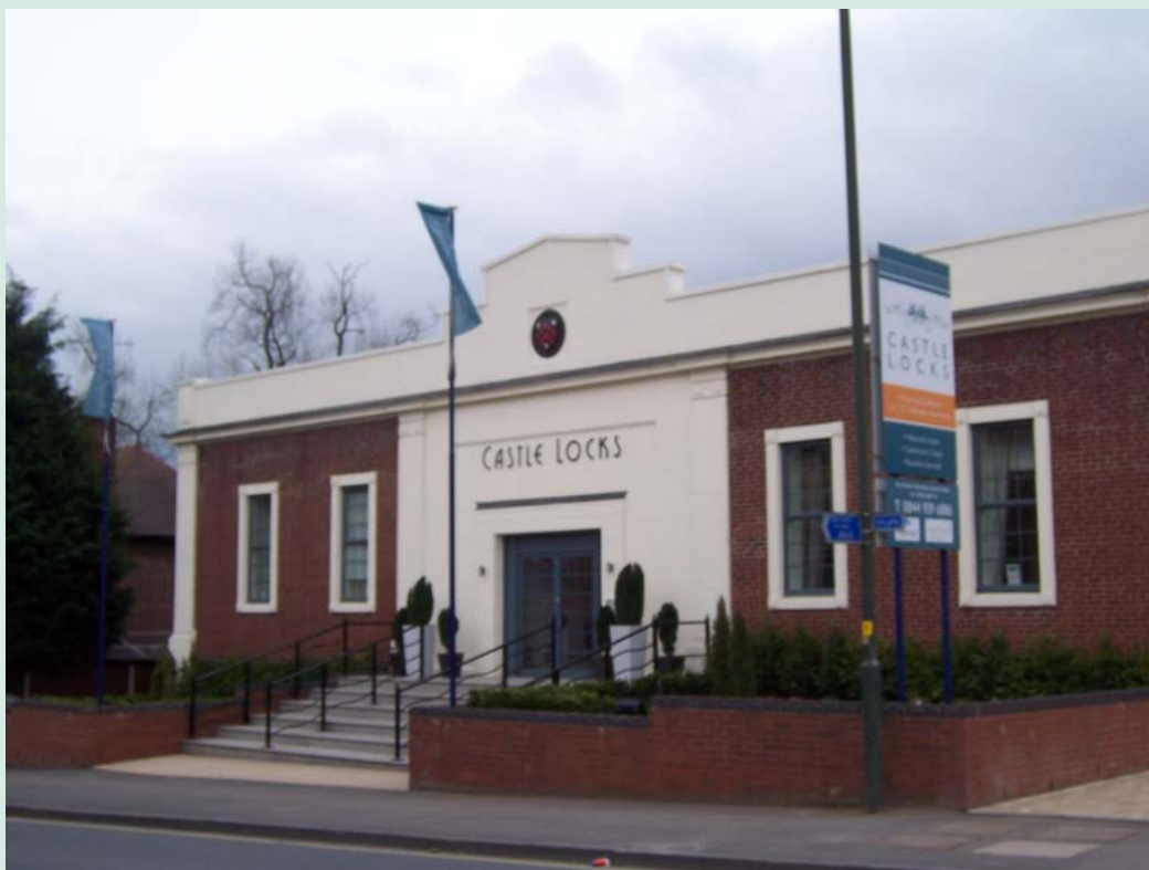
Castle Locks: Residential Development within Kidderminster Town Centre
