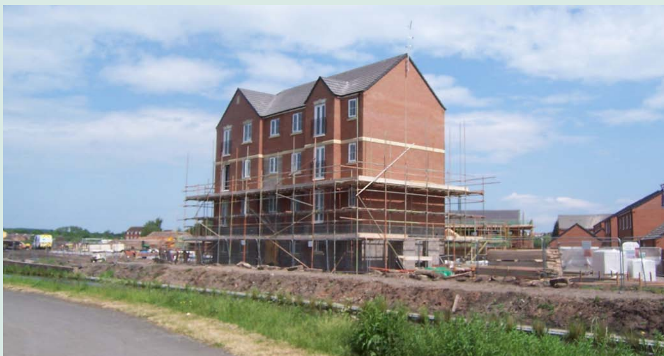
Canalside Apartments under Construction, Churchfields
