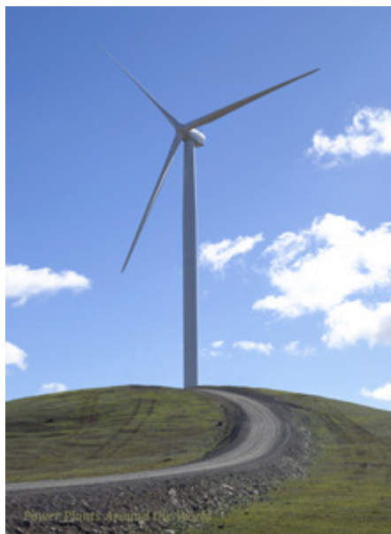
Figure 4 Horizontal Axis Wind Turbine (2.1 MW)
