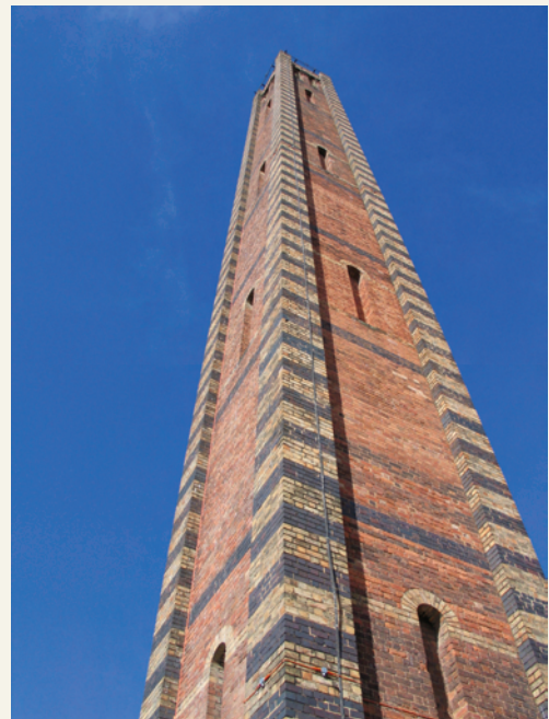
Chimney Stack, Weavers Wharf
