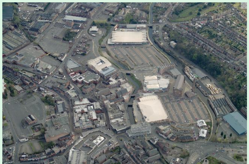
Surface car parks dominate the town centre
