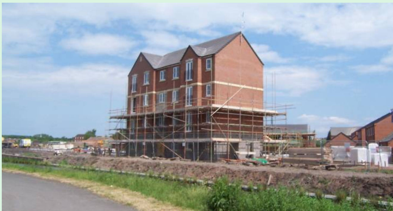
Canalside Apartments under Construction, Churchfields
