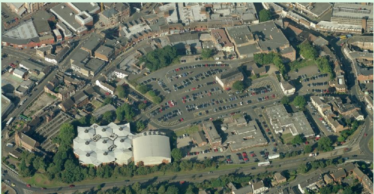
Aerial photo of Bromsgrove Street showing the fragmented urban fabric
