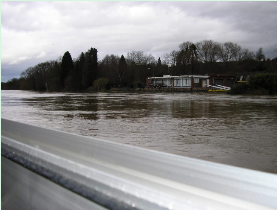
Flood Alleviation Scheme in Bewdley
