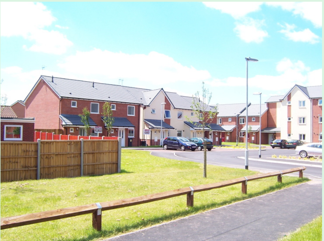
Affordable Housing, Stourport-on-Severn
