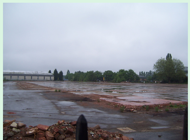
Former Rom Wire Site, Stourport Road, Kidderminster
