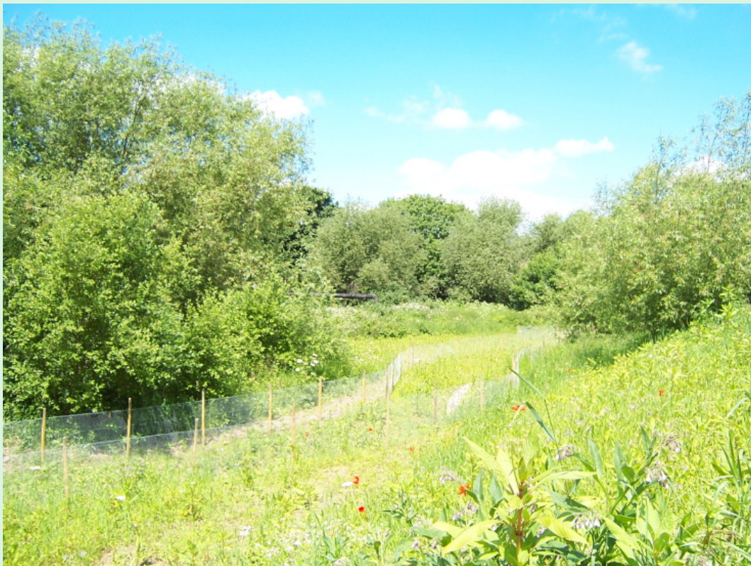
SUDS scheme in Stourport-on-Severn
