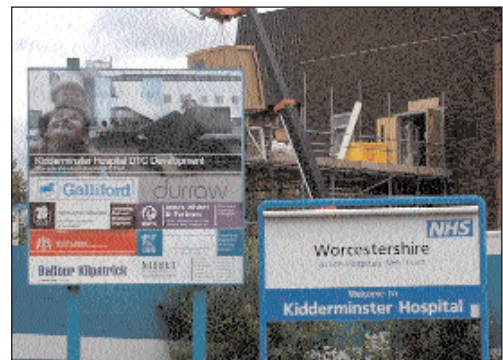
Construction of Diagnostic Treatment Centre, Kidderminster Hospital
