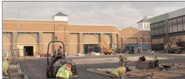
Weavers Wharf under construction
