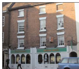
Flats above shops, Stourport-on-Severn
