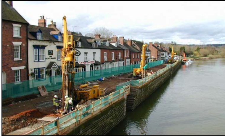
Implementation of flood defence barrier at Severnside North, Bewdley.
