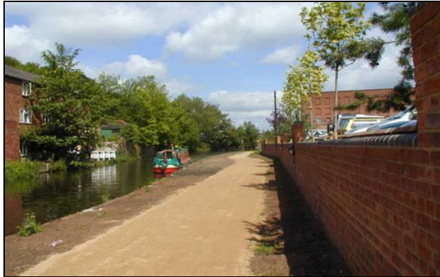
Improvements to Canal Towpath outside Tesco Store in Kidderminster
