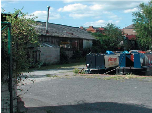
Rear of the STC.4 site viewed from Stroud Cruisers Boat Yard
