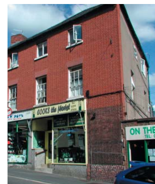
1b Bridge Street
