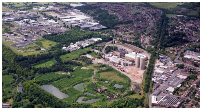
Aerial View of Stourport Road
