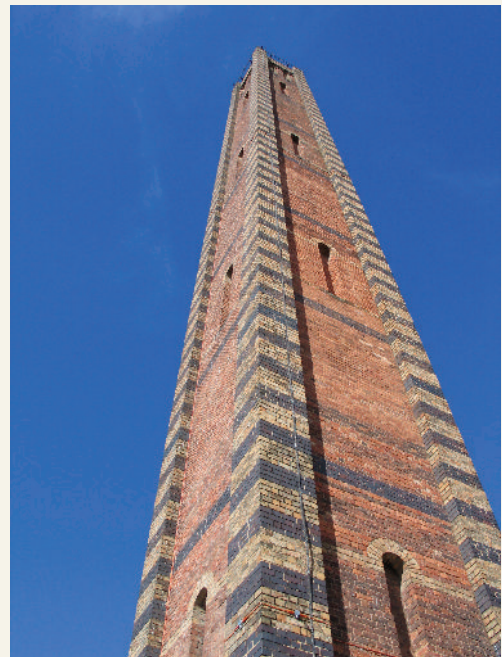
Chimney Stack, Weavers Wharf
