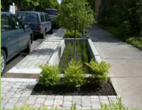
Combined rain garden and tree pit designed to receive run-off from the street. Photo credit: Dusty Gedge
