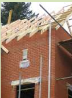
Bat tubes installed on new builds at Maybury Hill. Image courtesy of Taylor Wimpey and Ecosulis.
