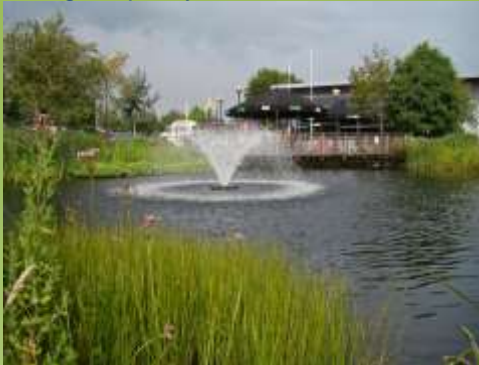
Hopwood Motorway Service Station; the environment here is designed to be attractive while also managing and cleaning (through the bioretention pond shown above) the waste and surface water run-off, prior to its discharge into local watercourses.
