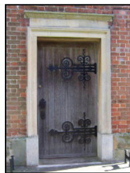
Principal door at St. Peter's Church
