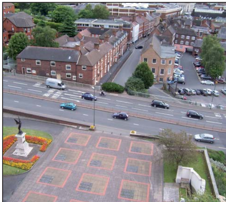
View of the Ring Road cutting across the north end of Church Street
