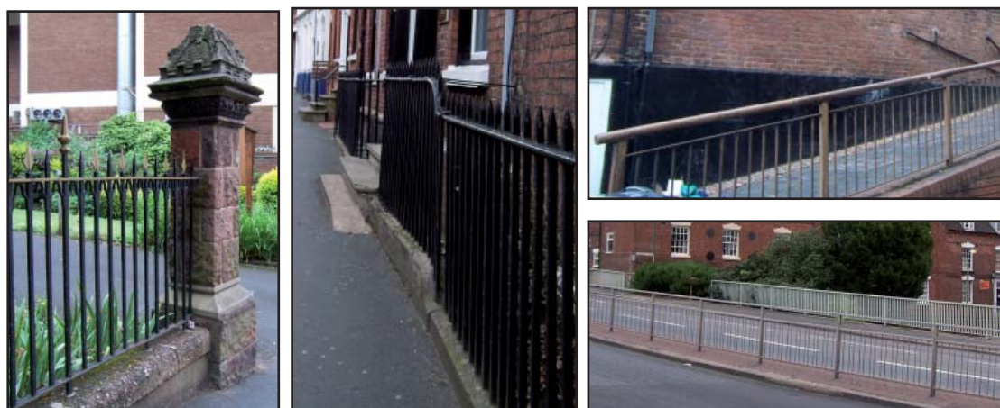
Examples of some of the types of railings present in the Area. Those on the left are traditional in character, those on the right are modern replacements or additions and do not enhance the overall appearance of the Area
