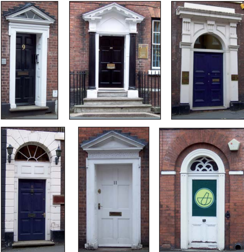
Example of types of doors and their surrounds found within the Area
