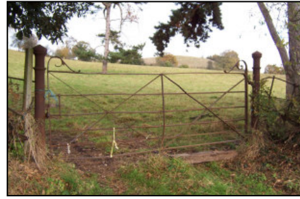
The survival of architectural features contribute to the character of the Area
