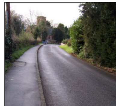
Standard tarmacadam used for both the road and pavement
