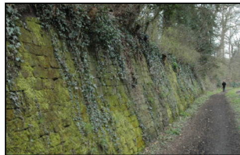
Old Forge Cottage retaining wall, Wolverley
