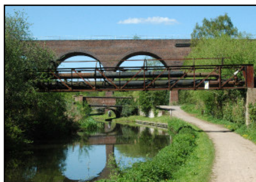
Severn Valley Railway Viaduct, Kidderminster
