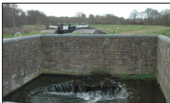
Wolverley Court lock and overflow
