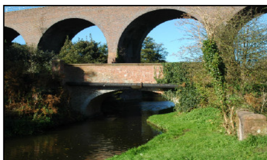
Falling Sands Bridge & Severn Valley Railway Viaduct
