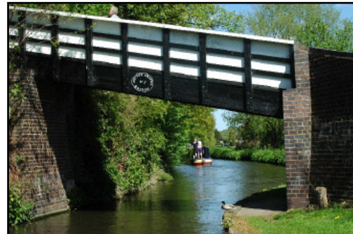
Mitton Chapel Bridge (no.7)
