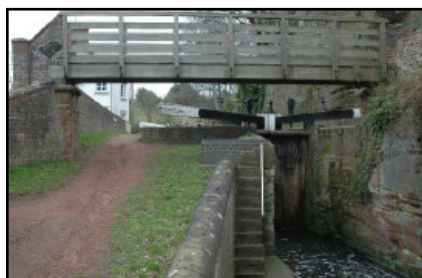
Debdale lock, bridge and house
