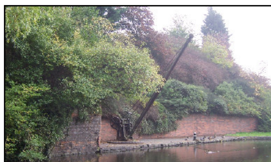
St Mary's crane and bollards
