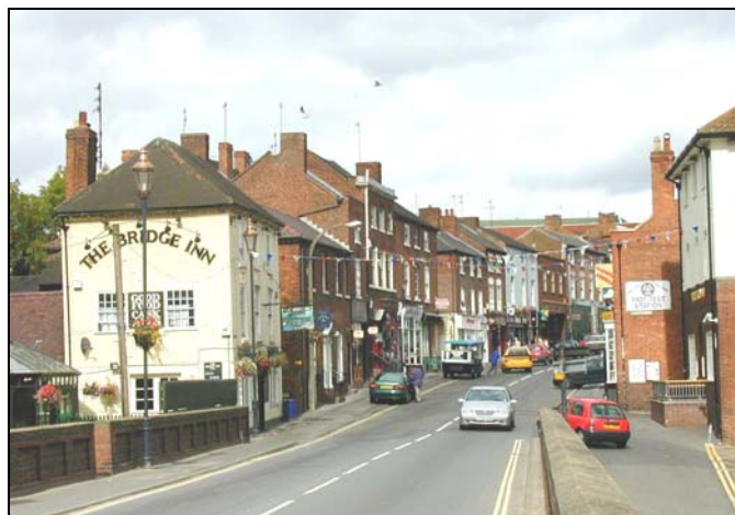
Stepped roofline in Bridge Street
