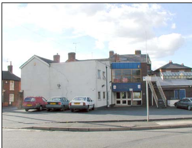
Extension to the rear of Nos. 9 & 10, Lichfield Street
