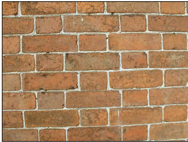
Brick-work with a traditional Flemish bond
