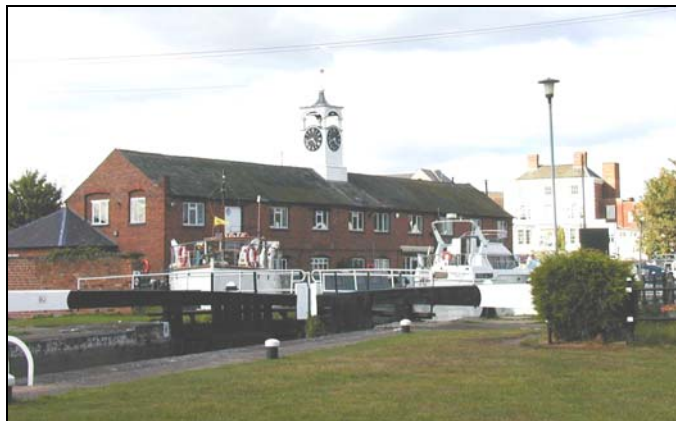
Former warehouse at the centre of the basins, now occupied by Stourport Yacht Club
