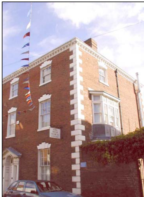
Quoins to the corner of a building in York Street
