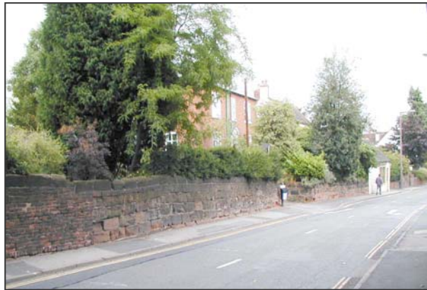
Sandstone walls in Mitton Street
