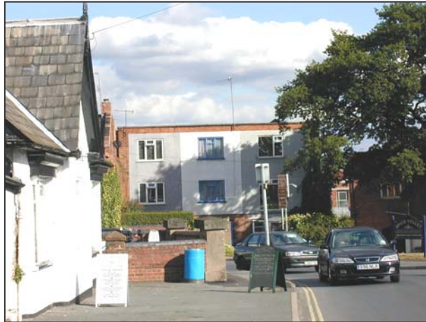
View looking east along York Street towards unsympathetic flat roofed houses in Lion Hill
