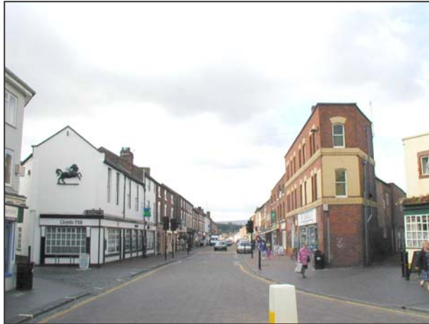
End profiles of buildings adjoining Parkes Passage (left) and Swan Passage (right)
