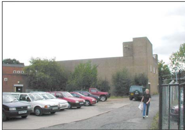
Unsympathetic rear elevations to buildings in High Street
