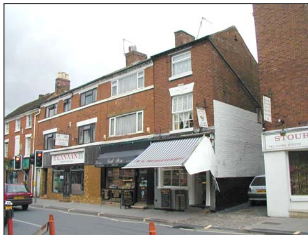
Replacement shop fronts and windows in York Street
