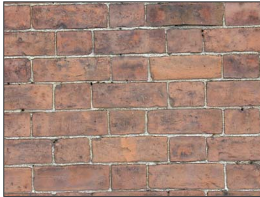
Brick-work with a traditional Flemish bond
