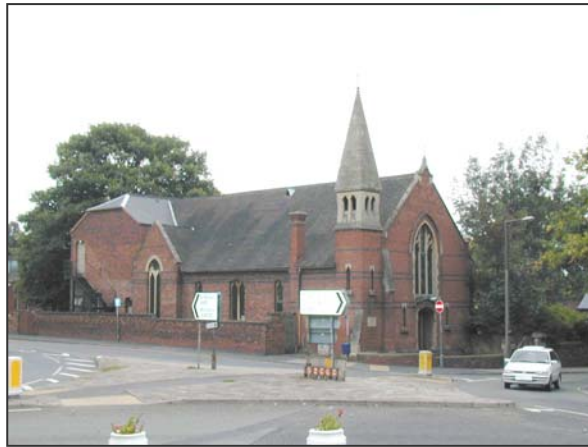
Church at the corner of Vale Road and Mitton Street
