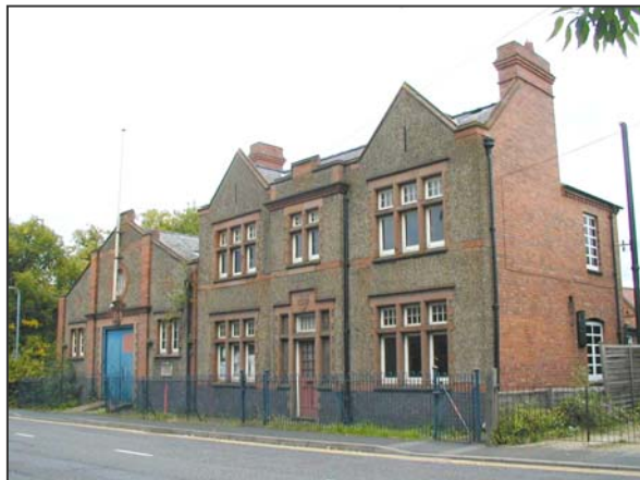
Former Army drill hall in Lion Hill
