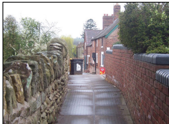
Examples of boundary walls within the Area
