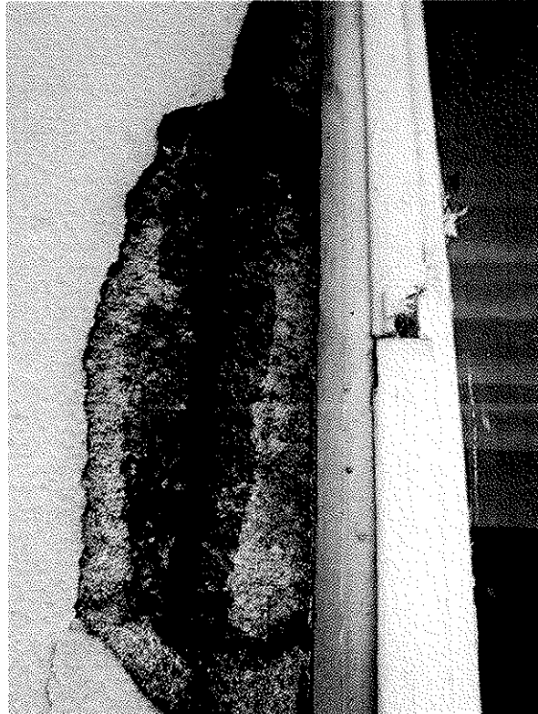
Photo 15: Detailed view showing an area of spalling with exposed reinforcement measuring 150x440x40 at the internal side elevation.
