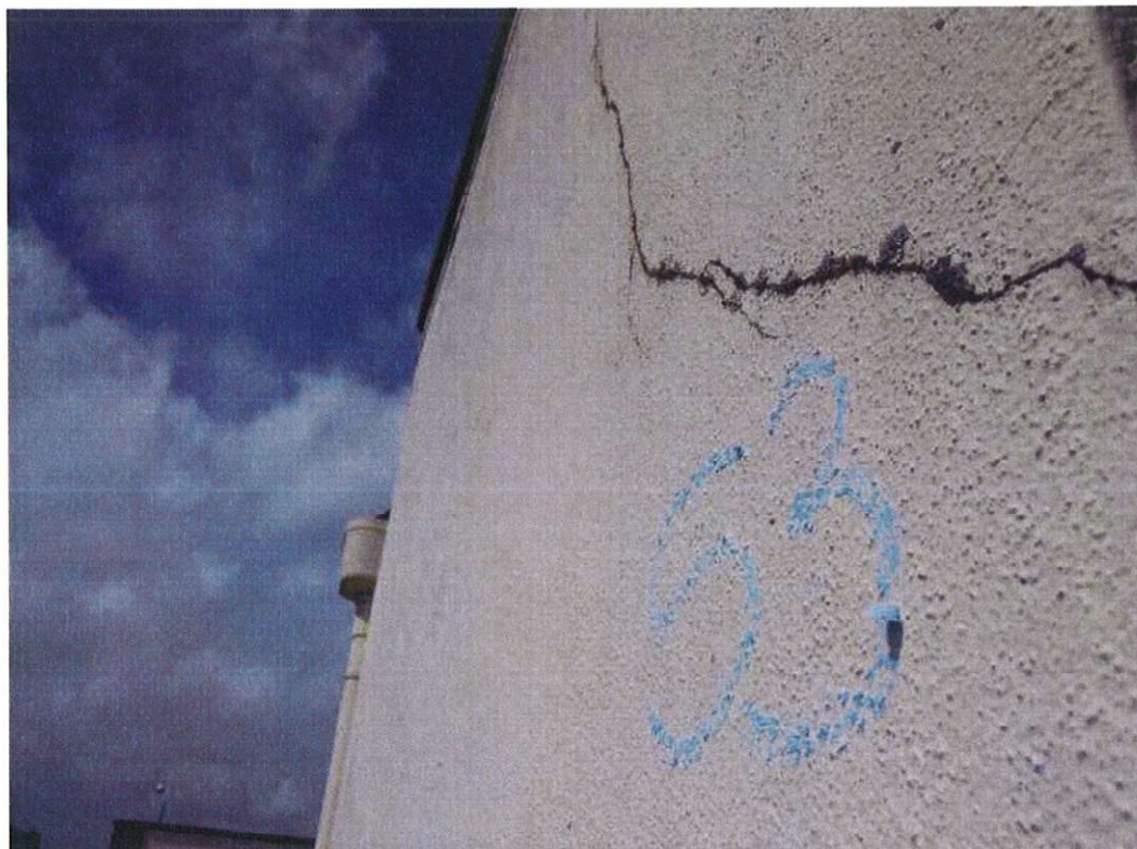
Photo 21: View showing a multi-directional crack measuring 500x1mm to side elevation D (Windermere Way).
