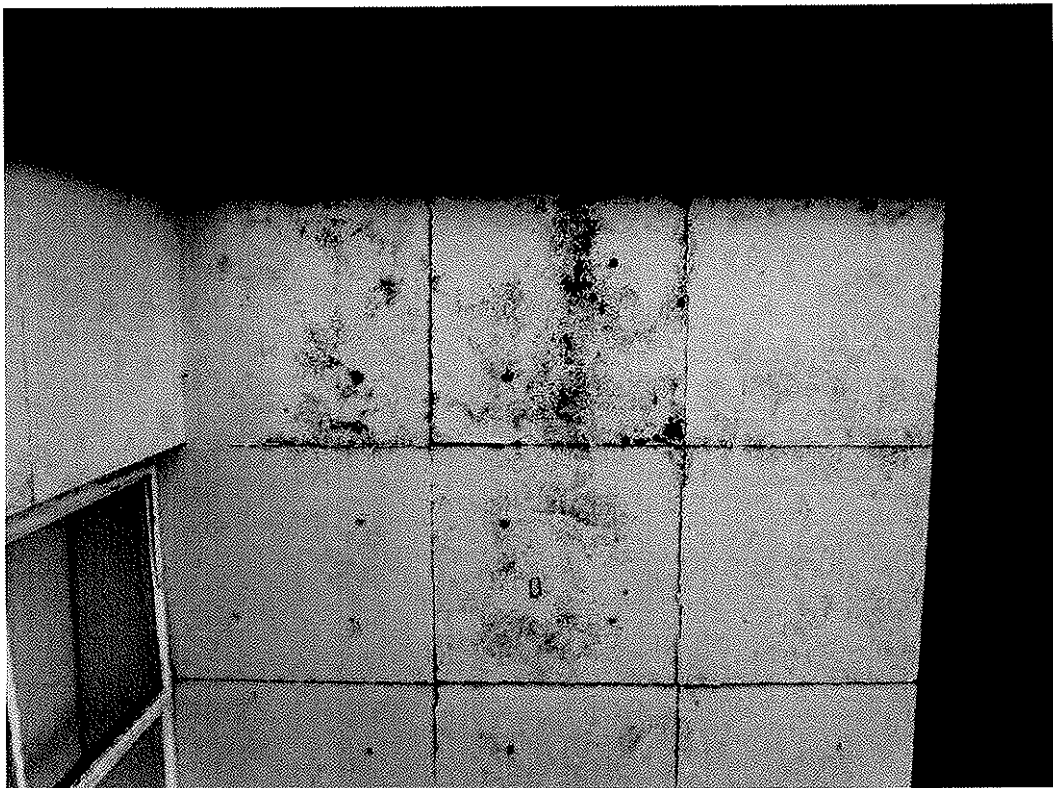
Photo 24: View showing paint flaking to front elevation C.
