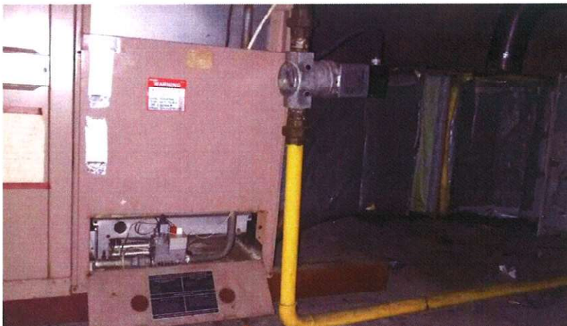
Drama block hot air heating plant
