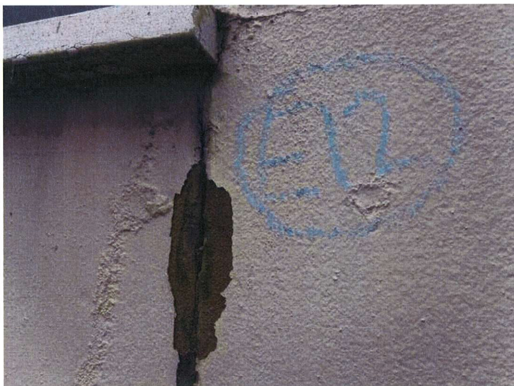
Photo 22: View showing joint mortar loss to the front elevation measuring 100x5x60mm.
