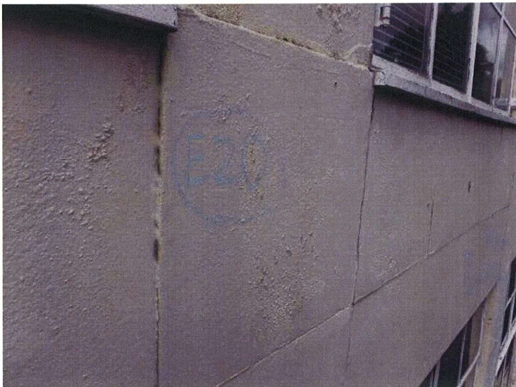
Photo 18: View showing a misaligned panel by up to 8mm on the front elevation, towards the south.
