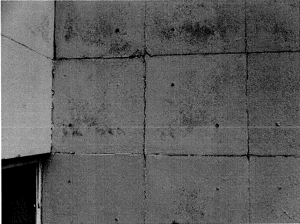
Photo 19: General view showing cracks to the paint at the panel joints typical throughout the structure.
