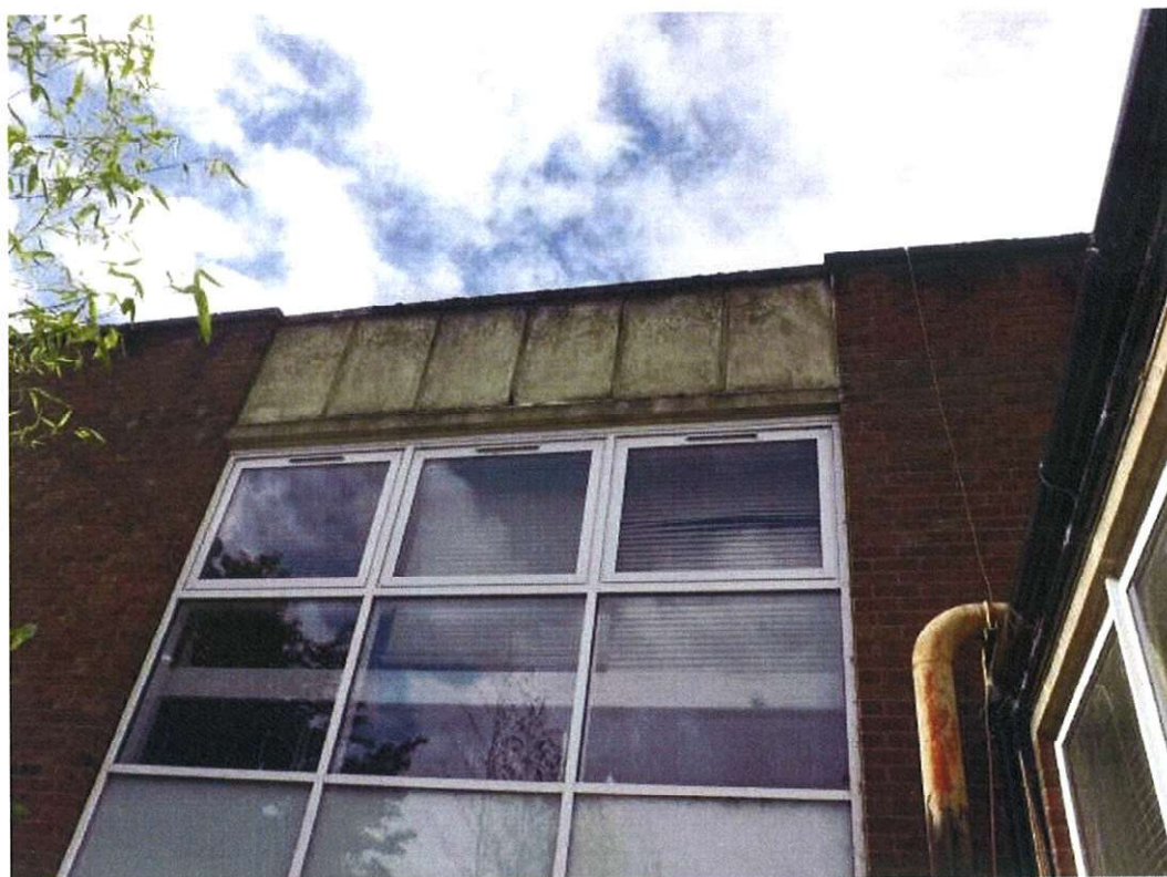
Photo 14: General view showing side elevation (Kingsway). Note the paint flaking.
