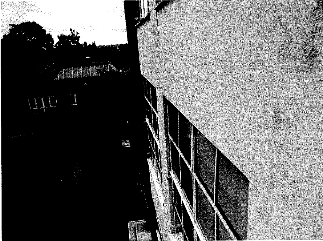
Photo 23: General view showing paint flaking at front elevation B, typical throughout the structure.
