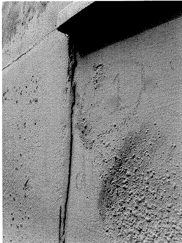
Photo 20: View showing a misaligned panel by 5mm to the front elevation which were typical throughout the structure.
