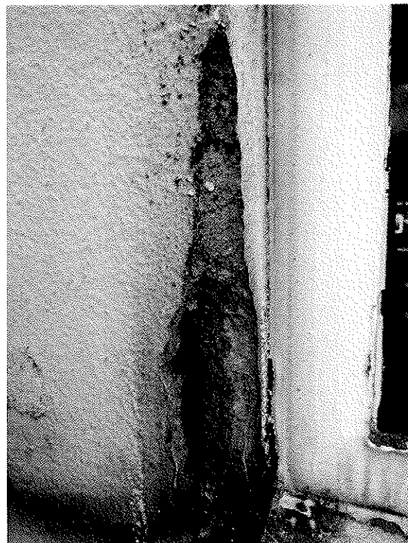
Photo 16: Detailed view showing an area of spalling with exposed reinforcement measuring 250x200x4mm at the internal side elevation.
