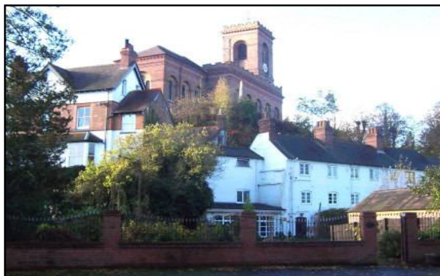
The position and size of the Church dominates the surrounding area
