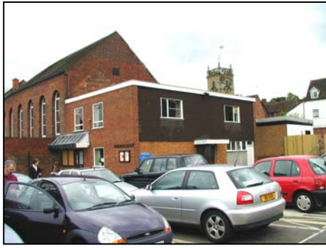
Extension to St. George's Hall (left) and lavatories to the rear of No. 69 Load Street (right)
