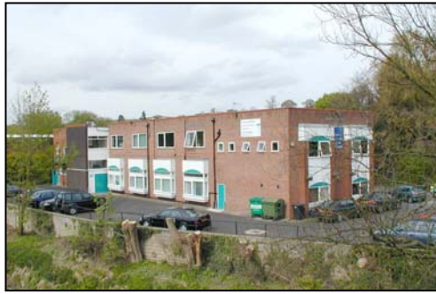
Bridge House adjoining the central bridge
