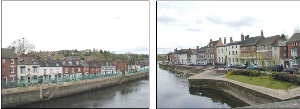
Severnside North (left) and Severnside South (right) from the central bridge
