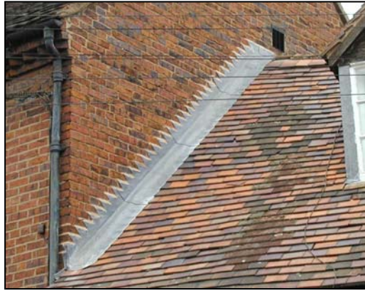
Lead flashing stepped with the mortar courses
