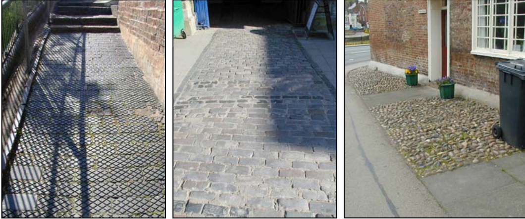
Traditional moulded setts (left) cut stone setts or cobbles (centre) and uncut pebbles or cobbles (right)
