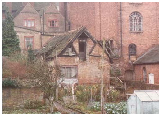
Outbuildings to the rear of Nos. 14 & 15, High Street
