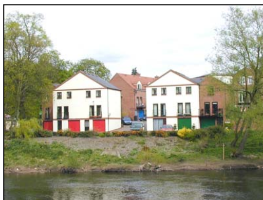
Riverside elevations of Millside Court, Wribbenhall. Note also the significant loss of riverside trees and exposure of soil
