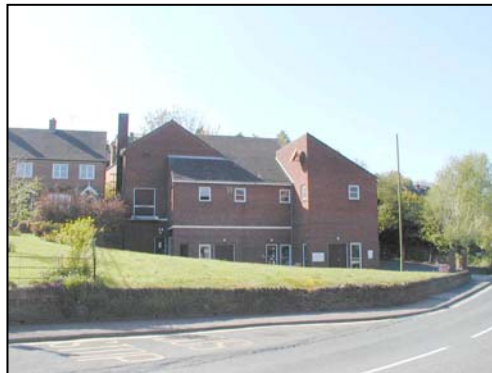
Telephone Exchange in Dowles Road
