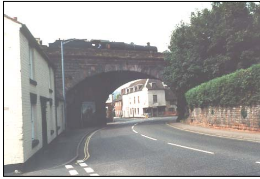
Viaduct over the Kidderminster Road
