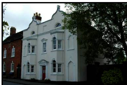
An example of polite architecture within the Area
