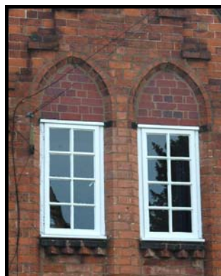
Poor quality and inappropriate features include Upvc window, glazed doors, and timber framing replaced with engineering brick.
