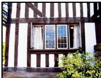
An example timber framing
