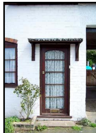
Poor quality and inappropriate features include Upvc window, glazed doors, and timber framing replaced with engineering brick.
