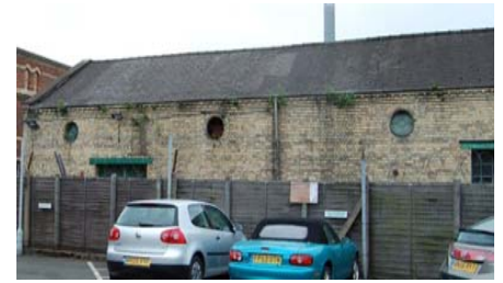
4: Green Street, Pumping Station and Sewage Works (former)
