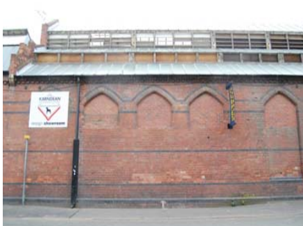
5: Green Street, Morton's Works (former)
