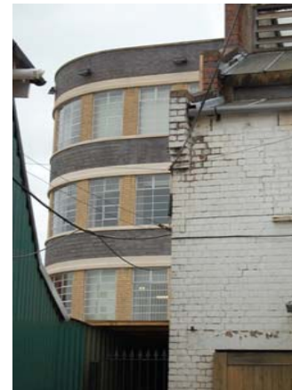
7: Off Dixon Street, view from courtyard of Morton's Works (former)
