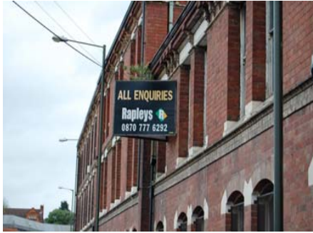
9: Green Street, Boucher's Works (former)
