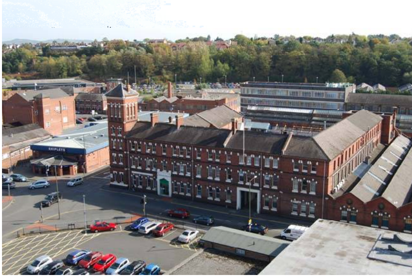
View looking east to Frank Stone, Elgar House and Morton's Works
