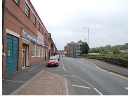
2: Green Street, gap
