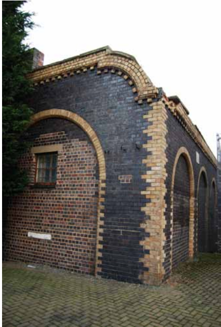
Perimeter Wall former Long Meadow Mills
