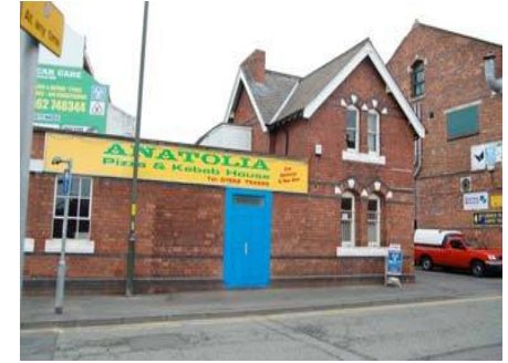
4: Dixon Street, dominant signage
