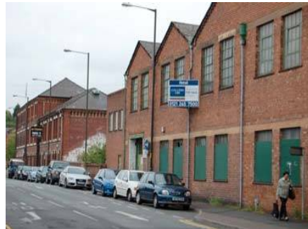
6: Green Street, Frank Stone (former) and Boucher's Works (former)
