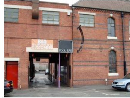
3: Off Green Street, Morton's Works (former)
