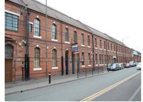
4: Green Street, Morton's Works (former)
