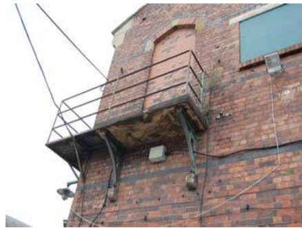
6: New Road, courtyard of Morton's Works (former)
