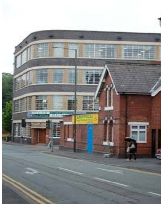
9: Green Street / Dixon Street, Victoria Carpet 10 (former), Elgar House
