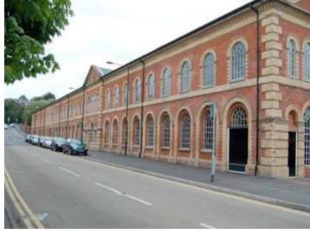
10: Green Street, Stour Vale Mill (former)
