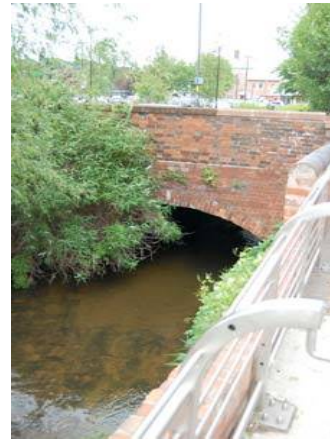
11: Green Street, Stour Vale Bridge
