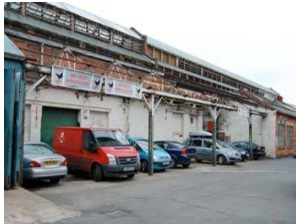
7: Green Street, Courtyard to Morton's Works (former)
