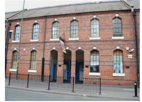
4: Green Street, Morton's Works (former)
