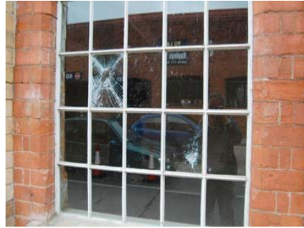
10: Green Street, Stour Vale Mill (former)
