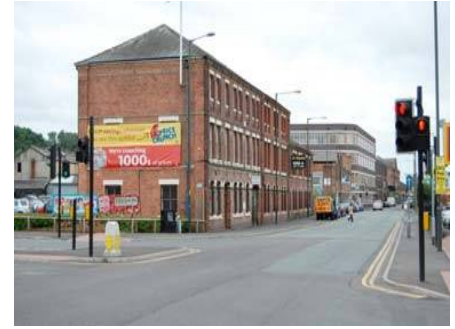
12: Green Street, looking south towards Boucher's Engineering Works (former)
