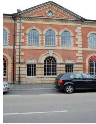
11: Green Street, Stour Vale Mill (former)
