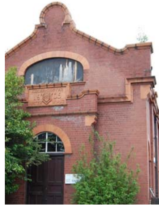
3: Pump Street, Pumping Station
