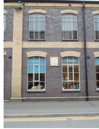
3: Green Street, Victoria Carpet 10 (former)
