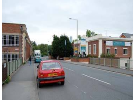
3: Castle Road, from Park Lane
