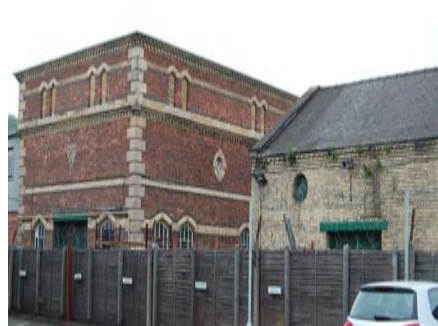
6: Green Street, Pumping Station and Sewage Works (former)
