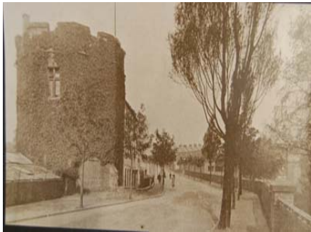
5: Castle Road, Caldwell Hall from east
