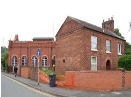
5: New Road / Pump Street, houses and Pumping Station
