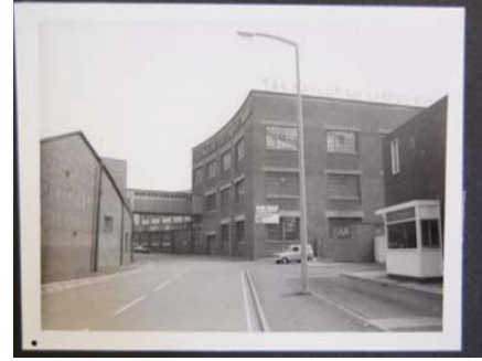
11: Green Street, bridge across from Naylors Ltd (former)
