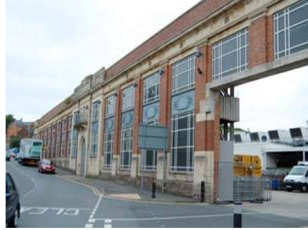
2: Castle Road, Brintons Works (former)
