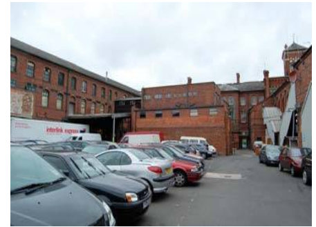
8: New Road, Courtyard of Morton's Works (former)
