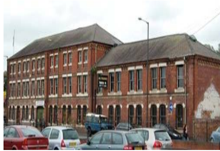
10: Green Street, Boucher's Engineering Works (former)
