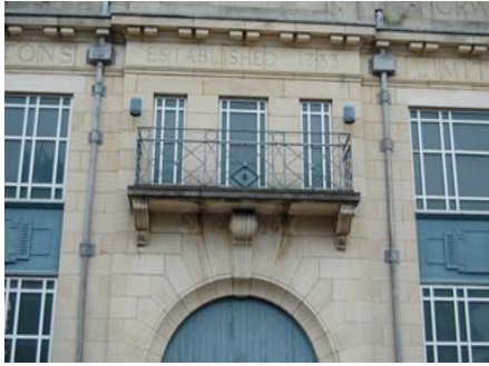
1: Castle Road, Brintons Works (former)
