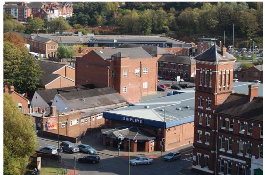
View looking east to Stourvale Mills, Boucher building and Morton's Works
