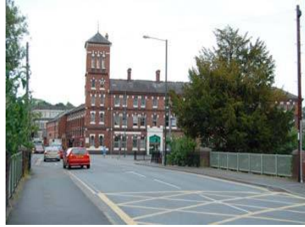
2: Castle Road, looking east towards Morton's Works (former)
