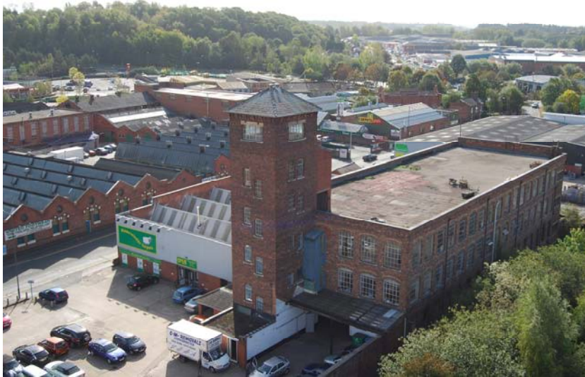
View looking south-east to Morton's Works, Pumping Station and Castle Mills
