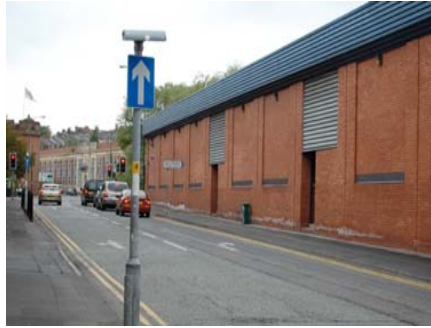
3: Dixon Street, intrusive structure
