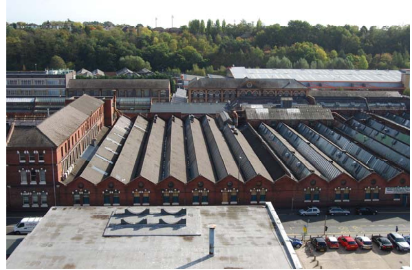
View looking east to Victoria Carpets and Morton's Works
