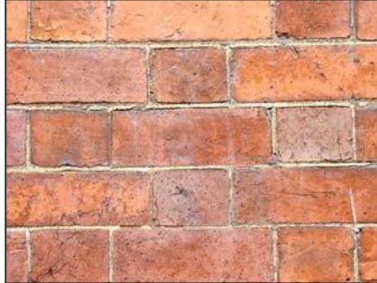
Brickwork with a Flemish bond
